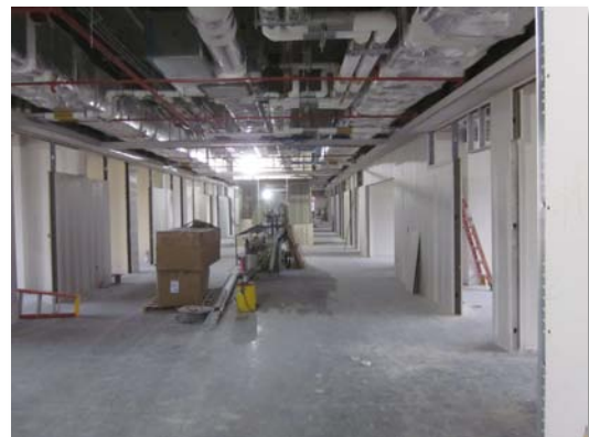
3 rd floor open office area and perimeter faculty offices.
