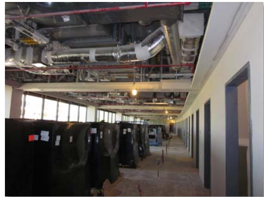
2 nd floor open lab with lab furniture ready for installation.
